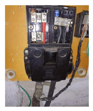
The ISCO cut-out example above shows a non-standard looped supply arrangement. The live loop to the neighbouring property is fed from the out-going terminals of the cut-out. When the fuse is withdrawn, the supply to both properties is de-energised.
