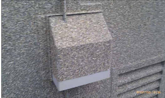
HINGED LOCK COVER CLOSED WITH PADLOCK ACCESS FROM BELOW AND ANTI JEMMY STRIPS TOP AND SIDES
