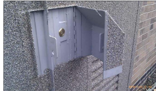
HINGED LOCK COVER OPEN SHOWING CLOAKED CYLINDER & PADLOCK HASPS ON DOOR AND COVER
