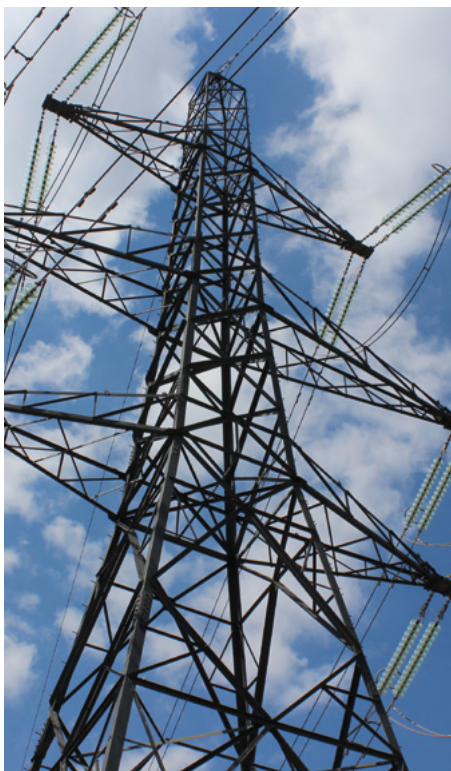
Figure 1: 275kV transmission line
