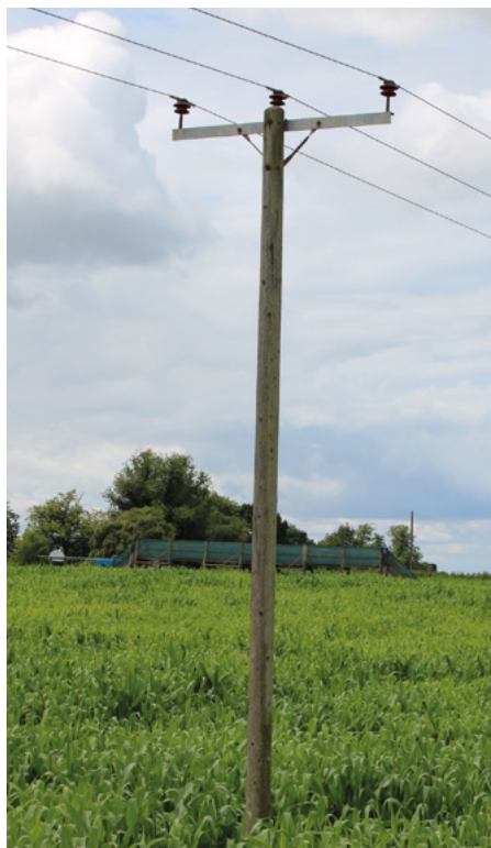
Figure 2: 11kV distribution line
