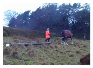
We swopped motor power for horsepower and used a heavy horse to remove wood poles that had supported overhead power lines from a rural area in South Yorkshire.
