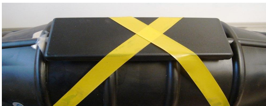
Figure 3 – Mark shell to indicate use of re-enterable resin
