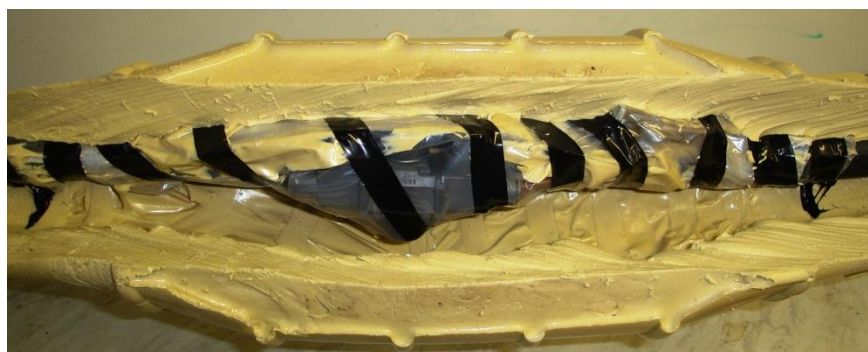
Figure 6 – Peel away resin to expose joint
