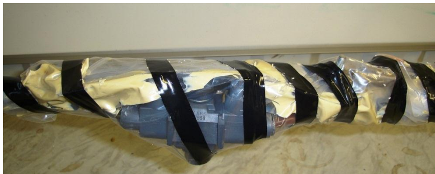
Figure 1 - Wrap joint in plastic bag
