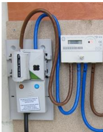
With polymeric/plastic incoming cable
