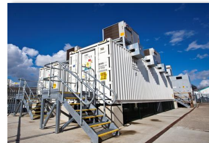
2.5MW battery at Rise Carr
